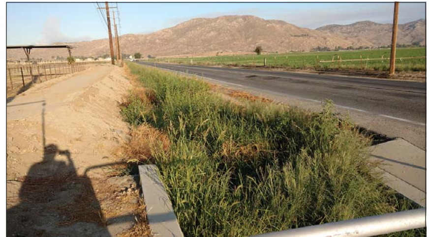
PHOTOGRAPH 8: Potential jurisdictional feature at the southwestern intersection of West Esplanade Drive and Cawston Avenue North.
