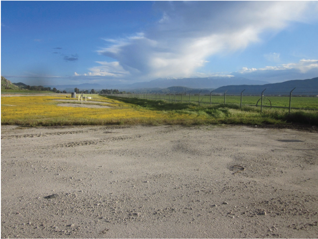
Overview of EM-25 Connection within fenced corridor (view to north)
