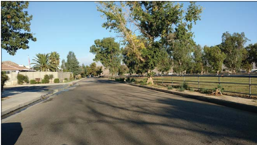
PHOTOGRAPH 7: Conditions along Commonwealth Avenue.
