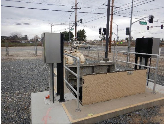
Photo 4.34-7 – Wet well exterior
