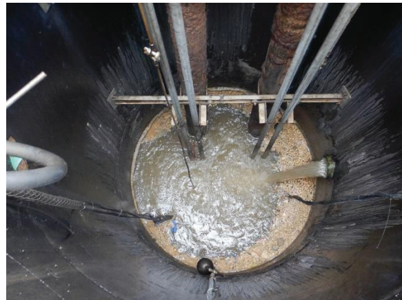
Photo 4.34-12 – Wet well interior (closeup)
