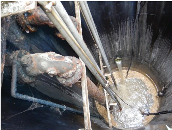
Photo 4.34-11 – Wet well interior (closeup)
