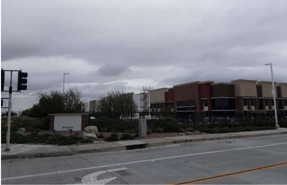
Photograph 7 View of P-33-019865, facing Northeast
