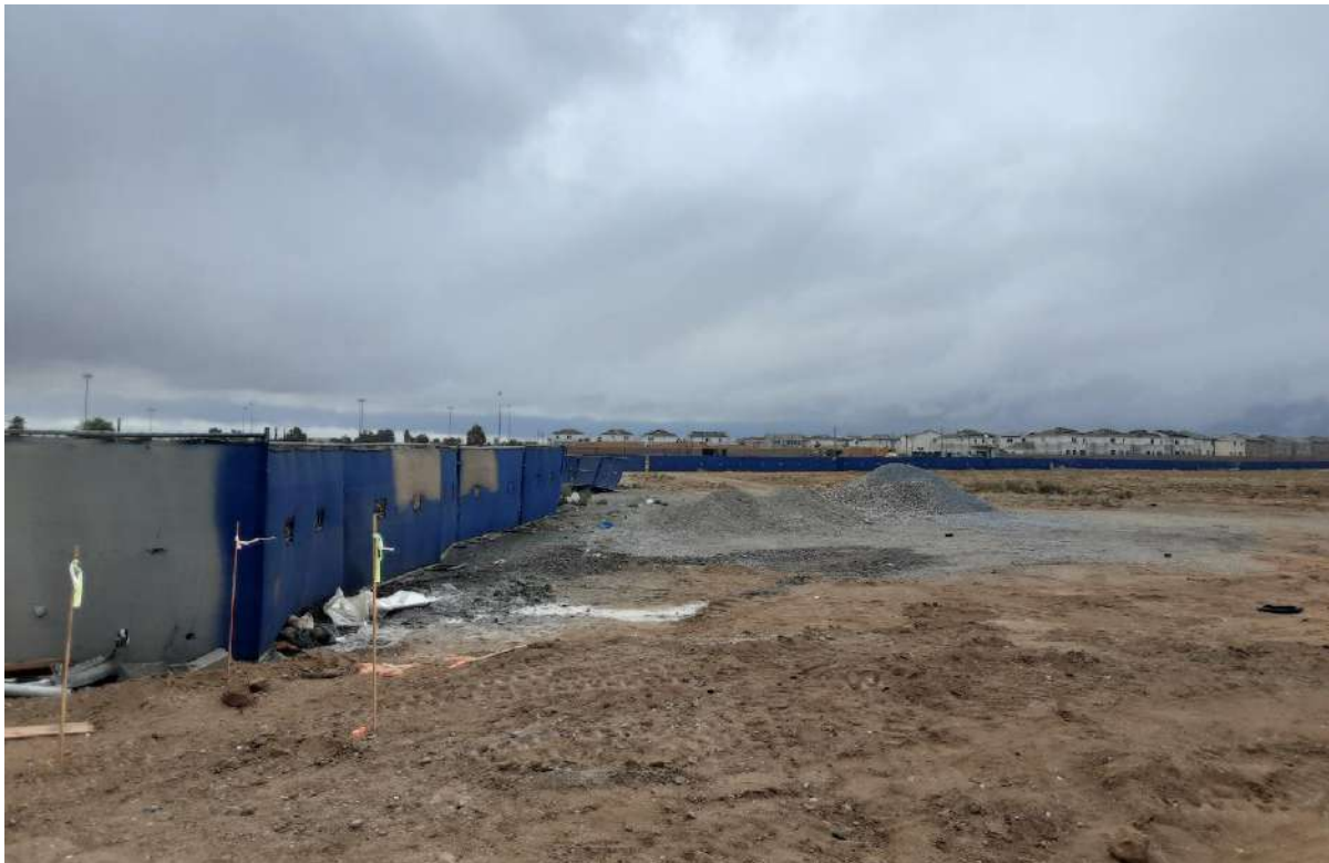
Photograph 8 View northwest of P-33-023936 showing blading and construction fencing
