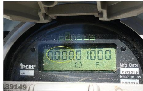
The 4 dials left to right appear on the water bill. The 4th dial is the first billing unit or BU. The leak indicator is the far right dial and will be advancing when water is being measured on the meter.
