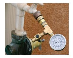
Using a pressure gauge, you can measure your water pressure at hose bibs in several areas, with and without water flowing inside the house. A drop in five (5) pounds of pressure is generally acceptable, any more can be a sign of a water pressure problem.
