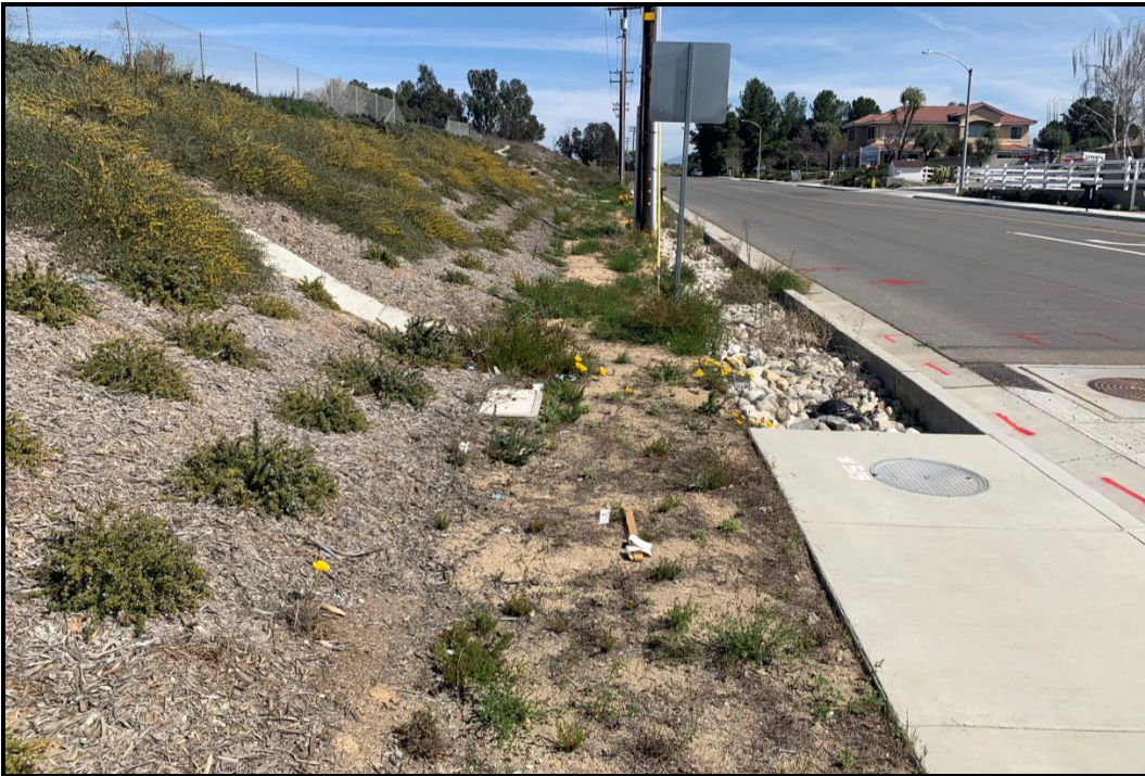
PHOTOGRAPH 1 North Side of Guava Street, Looking Northeast
