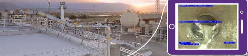
In 2022, EMWD added a new tool through a Closed Circuit Television system that allows it to identify areas with blockages, root intrusions, or other breaks in the sewer line so that corrective actions may be taken.
