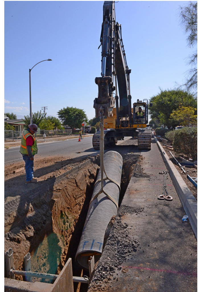
Phase 1 Feeder Construction
