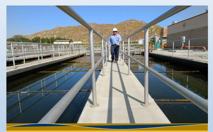
Employee Bill Walker, Moreno Valley Water Reclamations Operator Grade III, performing a walk inspection in the plant 's #1 secondary clarifier which is an inactive environment where solids are settled out prior to tertiary treatment
