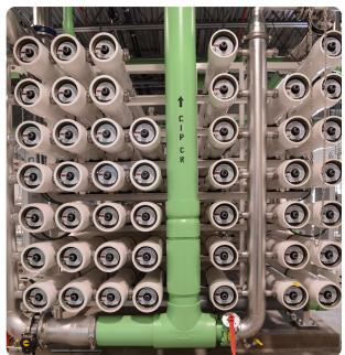
What is Desalination: EMWD uses groundwater desalination because the groundwater in the Perris and Menifee areas is salty. By removing the salts, we are making beneficial use of an otherwise unusable groundwater supply.
