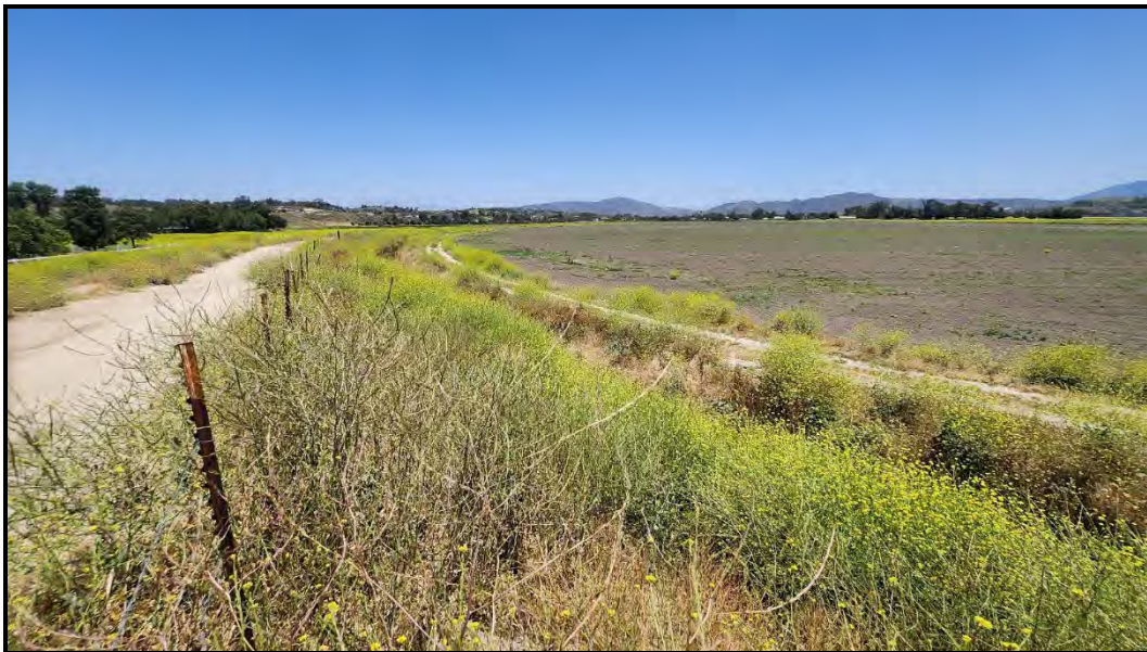
PHOTOGRAPH 6 View of Unlined Ditch South of an Unpaved Segment of De Portola Road, Facing Northeast
