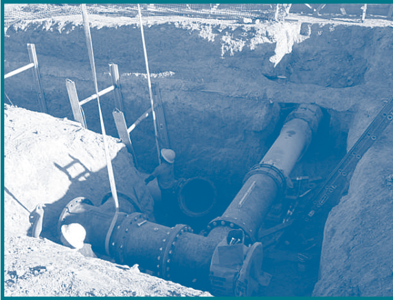
Perris Basin Desalination Facility under construction.
