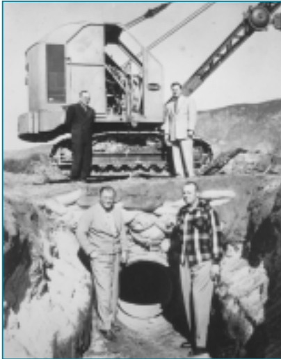
Eastern's early leaders inspect a pipeline under construction in 1953. Standing above, board member Irwin Farrar (left) and general manager Doyle Boen. In the trench are board members A.C. Messelheiser (left) and Johnny Kolb.
