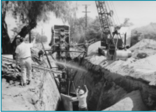
Trenching is hard work! Here, digging is underway to place a pipeline for the Hemet-San Jacinto regional sewer system in 1963.
