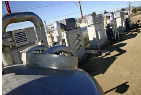
Fuel cells using digester gas at Moreno Valley Regional Water Reclamation Facility
