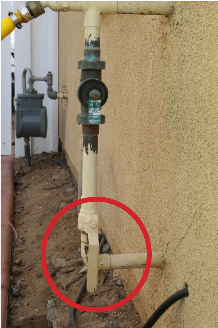
Water at house is "on"
