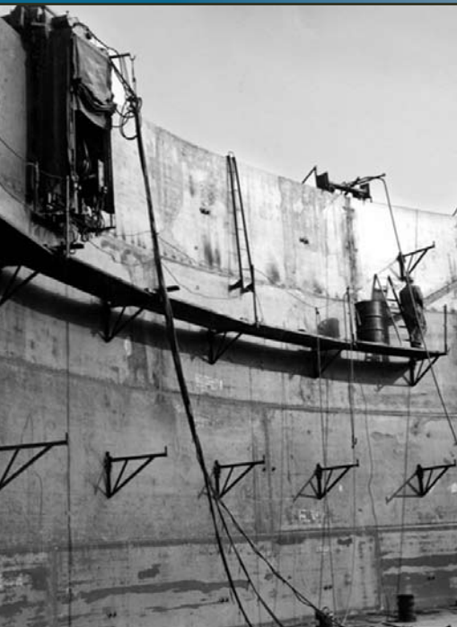
. 1960 CONSTRUCTION OF CHAMBERS TANK SERVING PERRIS AND SUN CITY
