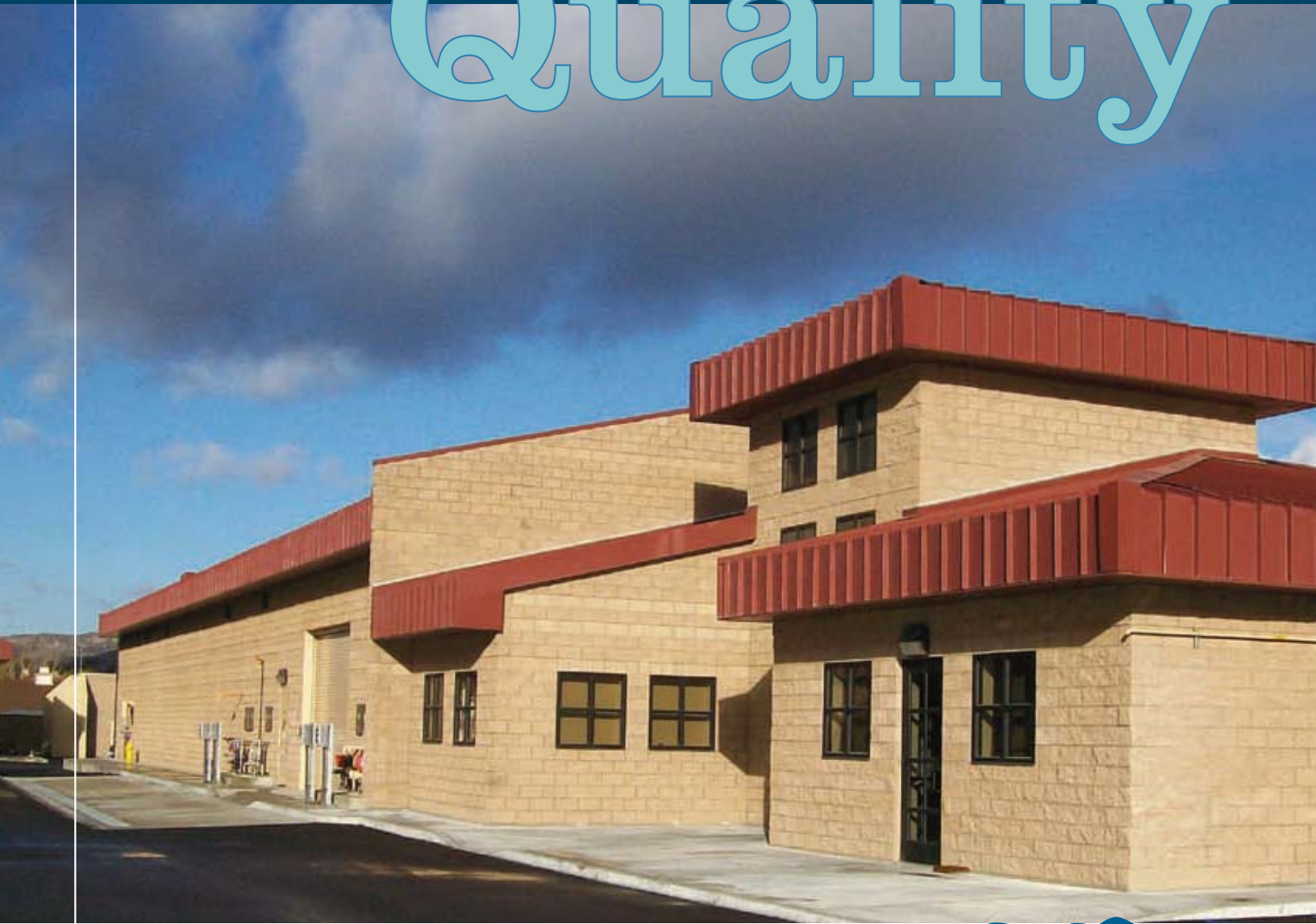
HEMET WATER FILTRATION PLANT
