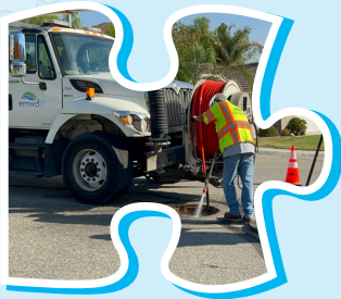
Preventative and predictive maintenance enables highly reliable operations.
