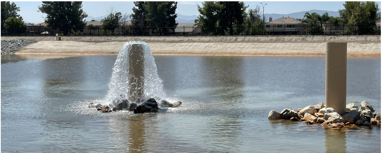
Mountain Avenue West Groundwater Replenishment Basins
