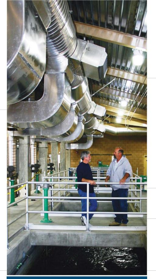
The Hemet Water Filtration Plant began service in 2006 using the latest membrane filtration to treat 10 million gallons a day. Over time, the plant's capacity will be increased to 40 million gallons a day.
