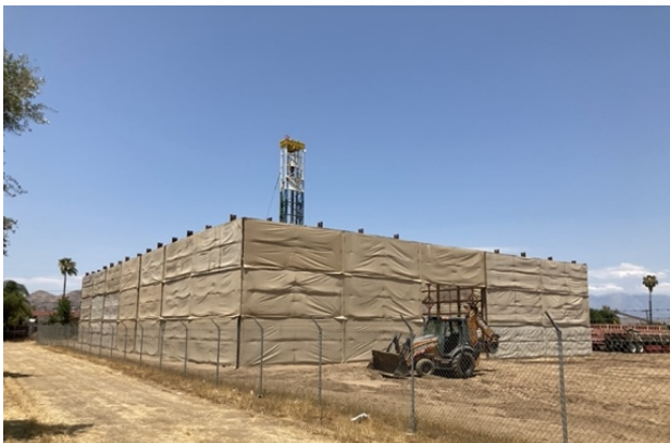
Sample of well drilling site with sound walls and drilling rig.
