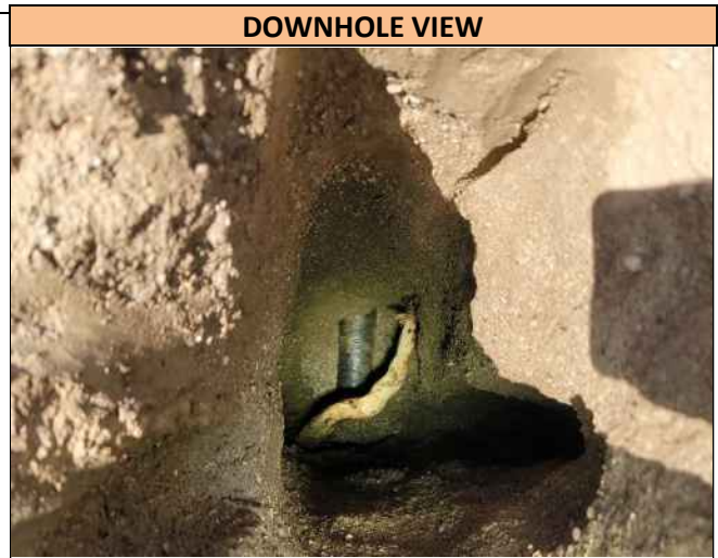
A downhole view of the 2.0 inch wide Steel Gas utility found in Pothole 8, at the depth of 44.0 inches T/P. Utility runs in a N/S direction at the Pothole location and was found directly on markout.
