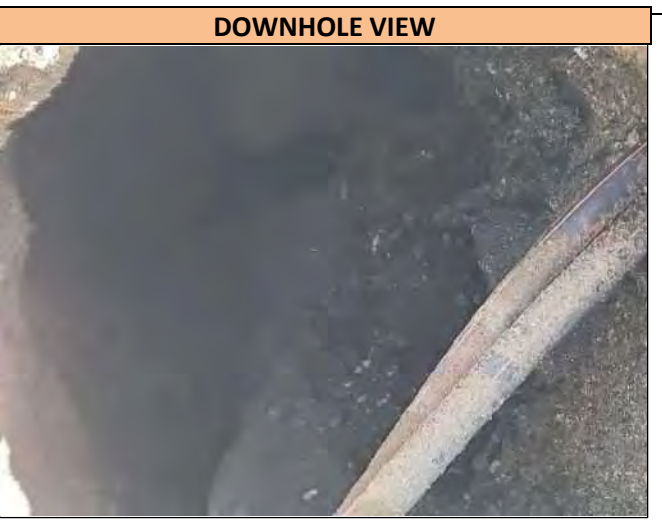
A downhole view of the two 1.0 inch wide Direct Bury Telecom utility found in Pothole 2, at the depth of 15.0 inches T/P. Utility runs in a SW&E direction at the Pothole location and was found directly on markout.
