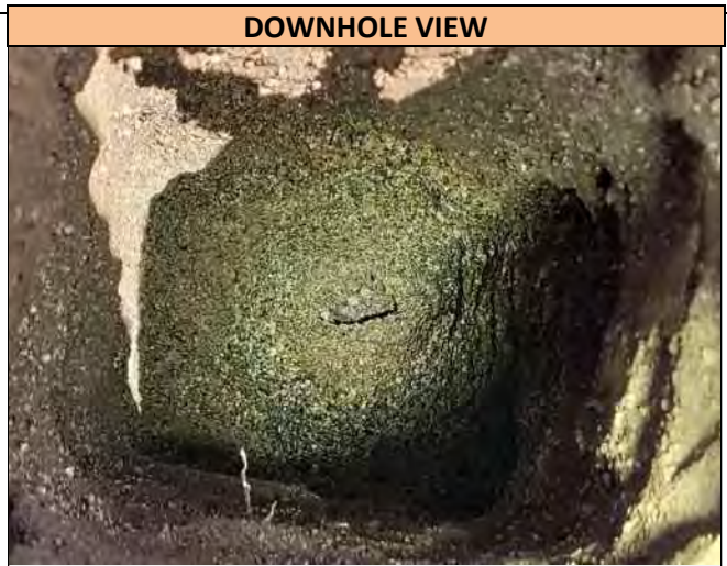
A downhole view of the excavation to 48.0 inches deep. Utilities were not found in the Pothole.
