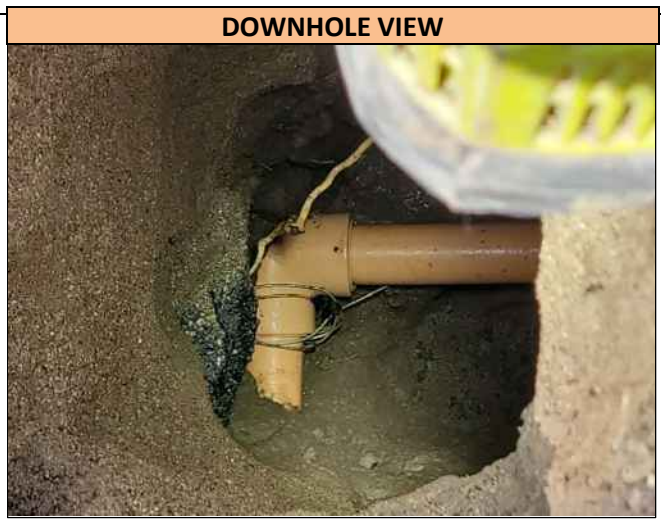
A downhole view of the 2.0 inch wide Plastic Gas T-connector utility found in Pothole 5, at the depth of 53.0 inches T/P. Utility runs in a N/S&E direction at the Pothole location and was found directly on markout.
