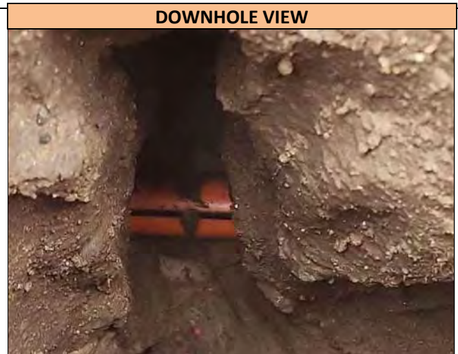
A downhole view of the 2.0 inch wide Plastic Fiber Optic, Telecom utility found in Pothole 22, at the depth of 37.0 inches T/P. Utility runs in a N/S direction at the Pothole location and was found directly on markout.
