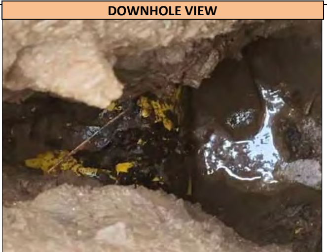
A downhole view of the 6.0 inch wide Steel Water utility found in Pothole 18, at the depth of 38.0 inches T/P. Utility runs in a N/S direction at the Pothole location and was found directly on markout.
