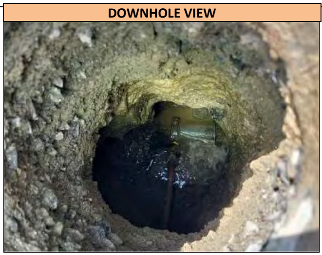
A downhole view of the utilities found in Pothole 23 and their orientation at the pothole location: 6.0 inch Steel Water utility at the depth of 59.0 inches T/P and runs in a WNW/ESE direction; and 1.0 inch Unknown Water utility at the depth of 57.0 inches T/P and runs in a NNE/SSW direction. Utilities were found directly on markout.
