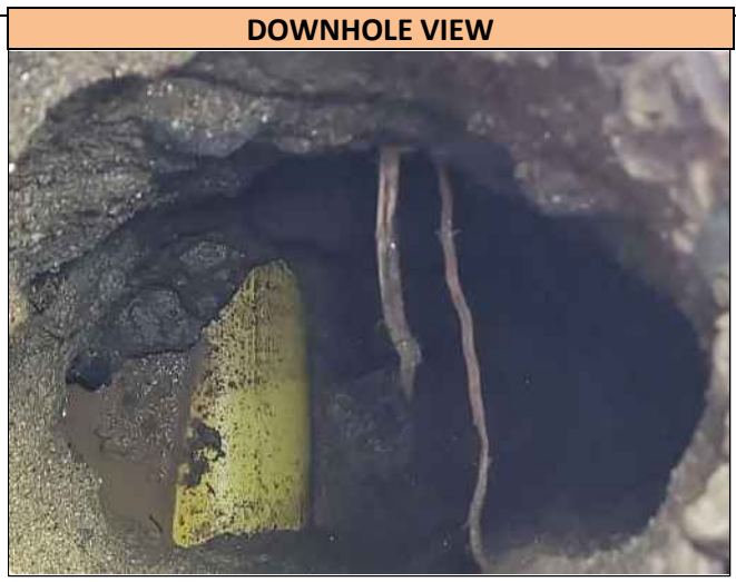
A downhole view of the 6.0 inch wide Plastic HP Gas utility found in Pothole 10, at the depth of 56.0 inches T/P. Utility runs in a W/E direction at the Pothole location and was found directly on markout.
