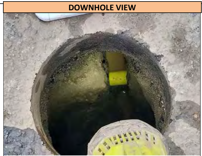
A downhole view of the 2.0 inch wide Plastic Gas utility found in Pothole 28, at the depth of 53.0 inches T/P. Utility runs in a N/S direction at the Pothole location and was found directly on markout.
