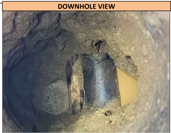
A downhole view of the 4.0 inch wide Steel Gas utility found in Pothole 11, at the depth of 43.0 inches T/P. Utility runs in a W/E direction at the Pothole location and was found directly on markout.
