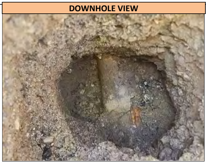
A downhole view of the 4.0 inch wide Concrete Water utility found in Pothole 15, at the depth of 26.0 inches T/P. Utility runs in a W&S direction at the Pothole location and was found directly on markout.
