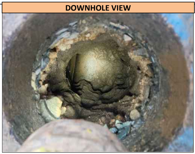
A downhole view of the 8.0 inch wide Steel Water utility found in Pothole 9, at the depth of 39.0 inches T/P. Utility runs in a N/S direction at the Pothole location and was found directly on markout.
