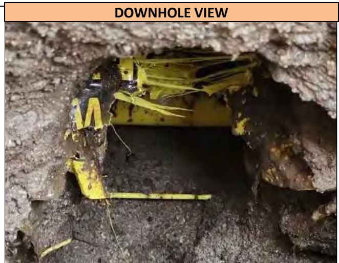
A downhole view of the 2.0 inch wide Plastic Gas utility found in Pothole 10, at the depth of 35.0 inches T/P. Utility runs in a N/S direction at the Pothole location and was found directly on markout.
