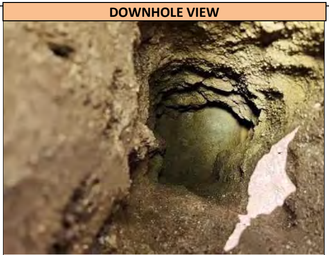
A downhole view of the 8.0 inch wide Concrete Water utility found in Pothole 18, at the depth of 44.0 inches T/P. Utility runs in a N/S direction at the Pothole location and was found directly on markout.
