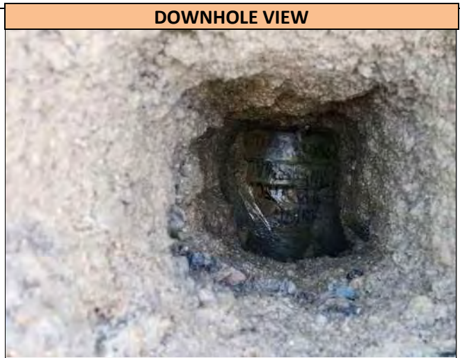
A downhole view of the 12.0 inch wide Steel Water utility found in Pothole 13, at the depth of 36.0 inches T/P. Utility runs in a W&SE direction at the Pothole location and was found directly on markout.
