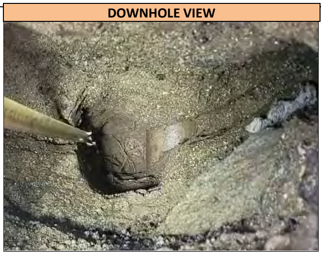
A downhole view of the 6.0 inch wide ACP Water utility found in Pothole 1, at the depth of 87.0 inches T/P. Utility runs in a N/S direction at the Pothole location and was found directly on markout.
