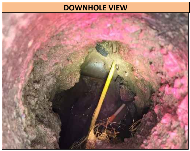
A downhole view of the utilities found in Pothole 26 and their orientation at the pothole location: 8.0 inch Steel Water utility at the depth of 53.0 inches T/P and runs in a WSW/ENE direction; 1.0 inch Plastic Gas utility at the depth of 36.0 inches T/P and runs in a NNW/SSE direction; and 1.0 inch Plastic Telecom utility at the depth of 49.0 inches T/P and runs in a NE/SW direction. Utilities were found directly on markout.
