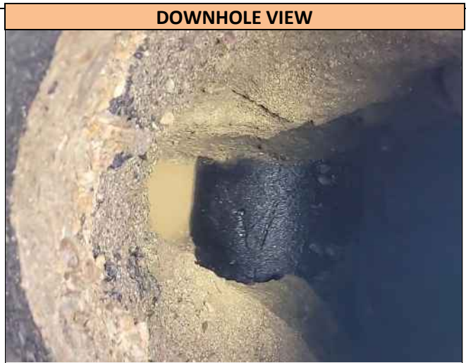
A downhole view of the 8.0 inch wide Steel Water utility found in Pothole 31, at the depth of 40.0 inches T/P. Utility runs in a N/S direction at the Pothole location and was found directly on markout.
