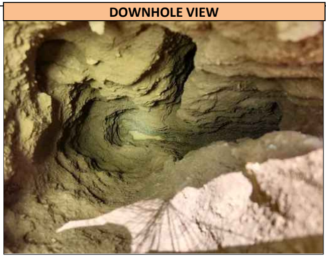
A downhole view of the excavation to 84.0 inches deep. Utilities were not found in the Pothole.
