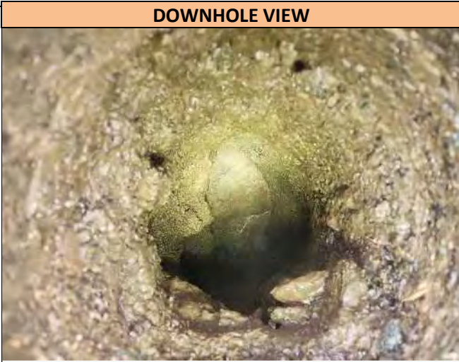
A downhole view of the 6.0 inch wide Concrete Water utility found in Pothole 12, at the depth of 33.0 inches T/P. Utility runs in a W/E direction at the Pothole location and was found directly on markout.
