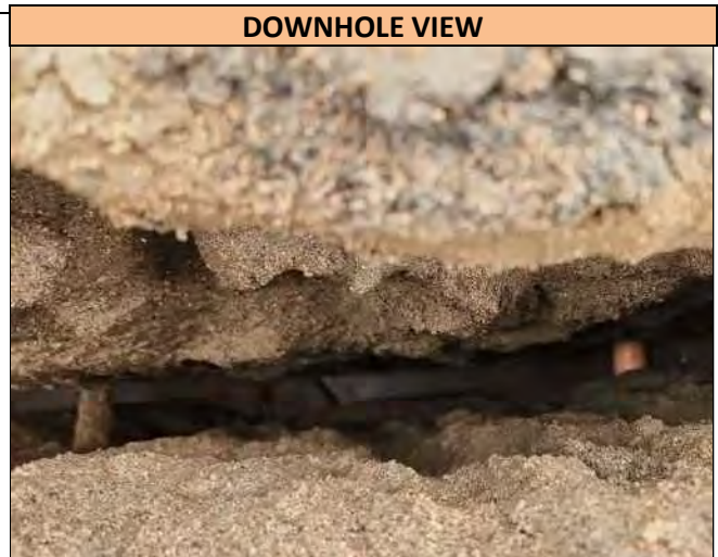
A downhole view of the 2.0 inch wide Plastic Gas utility found in Pothole 17, at the depth of 42.0 inches T/P. Utility runs in a N/S direction at the Pothole location and was found directly on markout.
