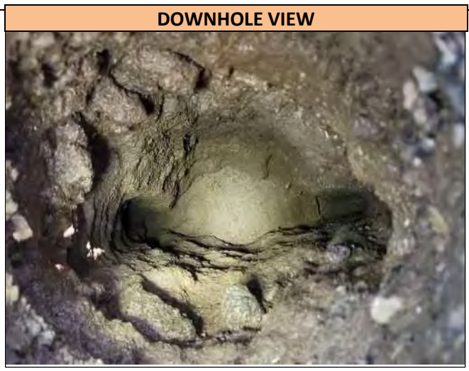
A downhole view of the 18.0 inch wide Concrete Water utility found in Pothole 12, at the depth of 56.0 inches T/P. Utility runs in a W/E direction at the Pothole location and was found directly on markout.
