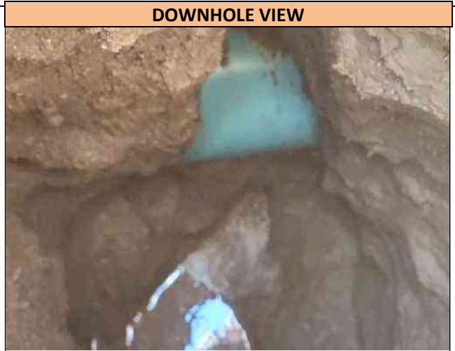
A downhole view of the 6.0 inch wide Plastic Water utility found in Pothole 16, at the depth of 47.0 inches T/P. Utility runs in a W/E direction at the Pothole location and was found directly on markout.
