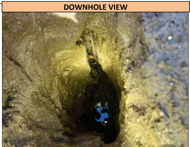
A downhole view of the 1.0 inch wide Copper Water Service utility found in Pothole 14A, at the depth of 47.0 inches T/P. Utility runs in a N/S direction at the Pothole location and was found directly on markout.
