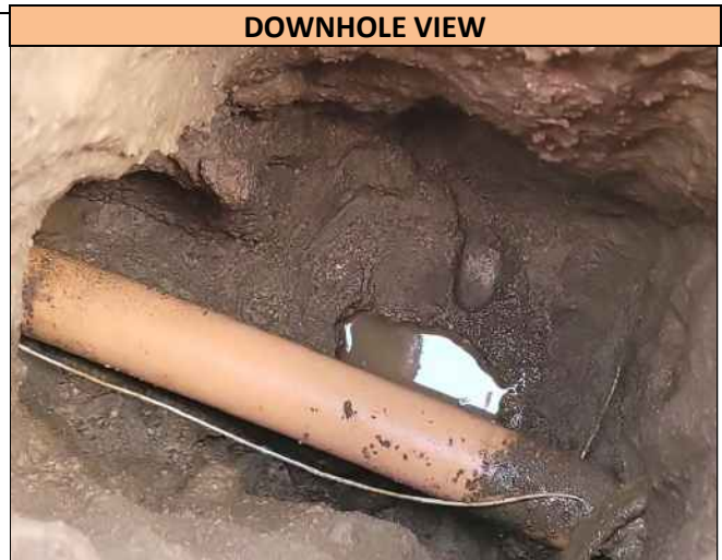
A downhole view of the 2.0 inch wide Plastic Gas utility found in Pothole 6, at the depth of 33.0 inches T/P. Utility runs in a W/E direction at the Pothole location and was found directly on markout.
