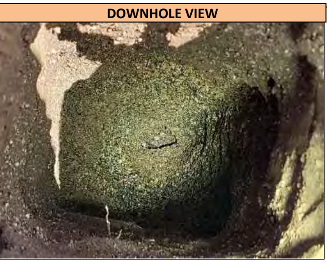
A downhole view of the excavation to 48.0 inches deep. Utilities were not found in the Pothole.
