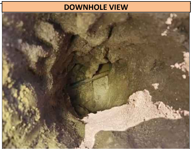
A downhole view of the 1.0 inch wide Direct Bury Telecom utility found in Pothole 21, at the depth of 30.0 inches T/P. Utility runs in a WSW/ENE direction at the Pothole location and was found directly on markout.
