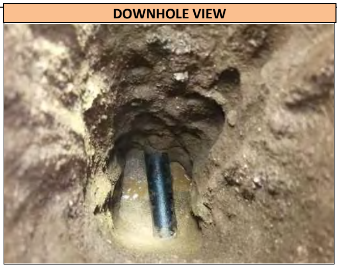
A downhole view of the 2.0 inch wide Steel Gas utility found in Pothole 22, at the depth of 33.0 inches T/P. Utility runs in a N/S direction at the Pothole location and was found directly on markout.
