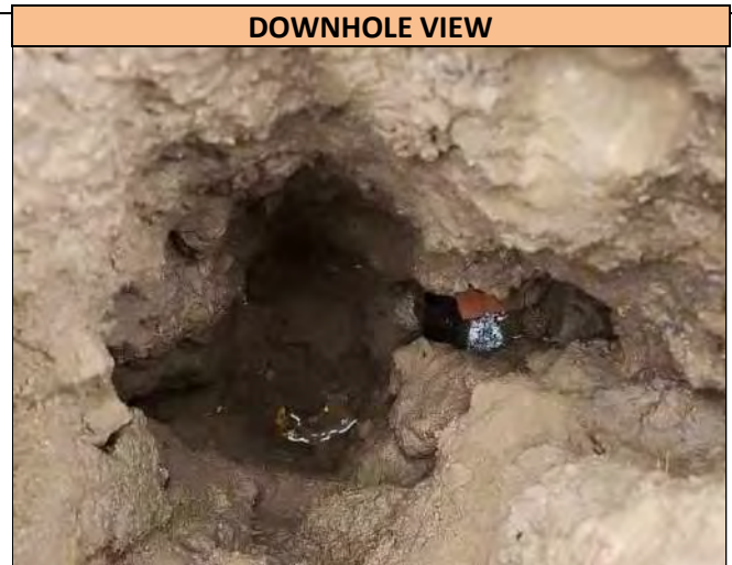
A downhole view of the 6.0 inch wide Steel Water utility found in Pothole 19, at the depth of 33.0 inches T/P. Utility runs in a W/E direction at the Pothole location and was found directly on markout.
