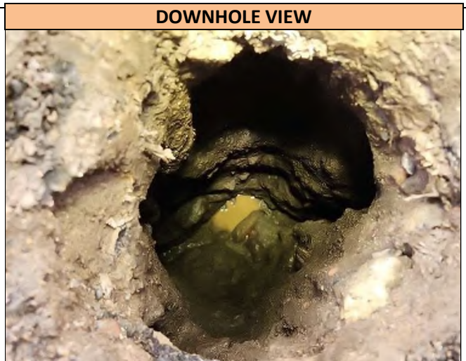
A downhole view of the excavation to 57.0 inches deep. Utilities were not found in the Pothole.
