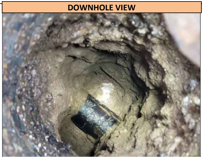
A downhole view of the 6.0 inch wide Steel Water utility found in Pothole 27, at the depth of 34.0 inches T/P. Utility runs in a N/S direction at the Pothole location and was found directly on markout.
