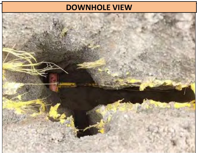
A downhole view of the utilities found in Pothole 13 and their orientation at the pothole location: 1.0 inch Plastic Gas utility at the depth of 44.0 inches T/P and runs in a W/E direction; and 3.0 inch Plastic Gas utility at the depth of 41.0 inches T/P and runs in a N/S direction. Utilities were found directly on markout.
