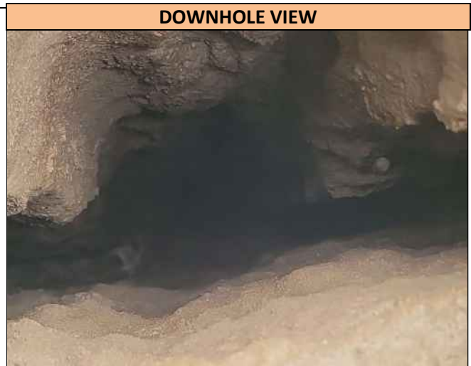
A downhole view of the excavation to 60.0 inches deep. Utilities were not found in the Pothole.
