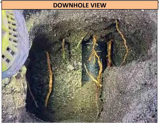
A downhole view of the 2.0 inch wide Steel Gas utility found in Pothole 5, at the depth of 30.0 inches T/P. Utility runs in a N/S direction at the Pothole location and was found directly on markout.
