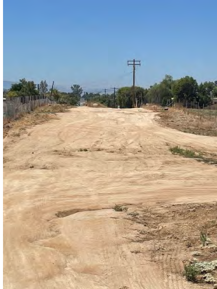
Photo 16: Facing east (Feature GH-02, 04).
