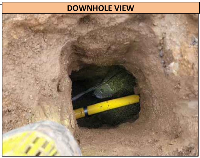
A downhole view of the 2.0 inch wide Plastic Gas utility found in Pothole 2, at the depth of 37.0 inches T/P. Utility runs in a W/E direction at the Pothole location and was found directly on markout.
