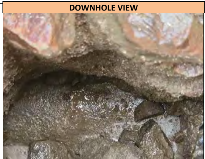
A downhole view of the 6.0 inch wide Concrete Water utility found in Pothole 11, at the depth of 36.0 inches T/P. Utility runs in a W/E direction at the Pothole location and was found directly on markout.
