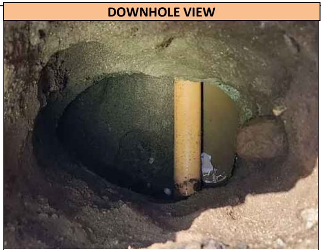
A downhole view of the 2.0 inch wide Plastic Gas utility found in Pothole 16, at the depth of 50.0 inches T/P. Utility runs in a WNW/ESE direction at the Pothole location and was found directly on markout.
