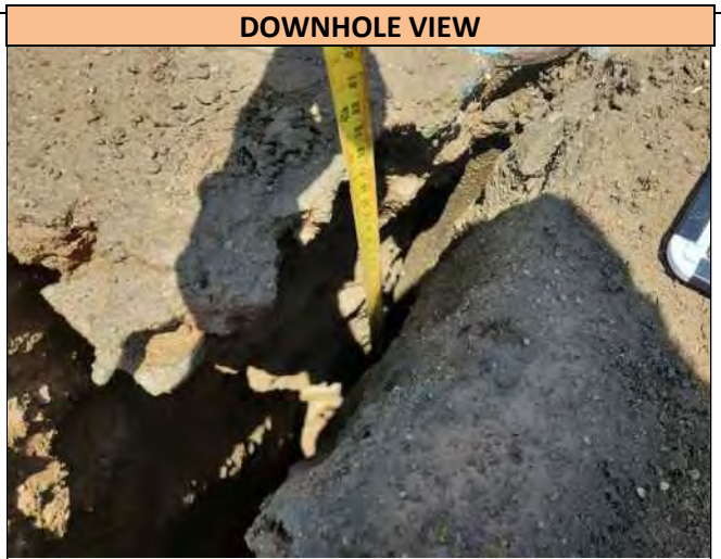
A downhole view of the 8.0 inch wide Steel Water utility found in Pothole 19, at the depth of 58.0 inches T/P. Utility runs in a N&W direction at the Pothole location and was found directly on markout.
