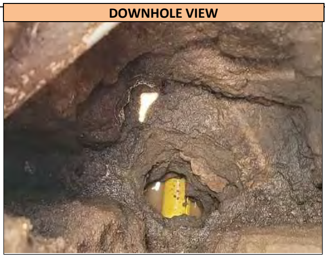
A downhole view of the 2.0 inch wide Plastic Gas utility found in Pothole 1, at the depth of 40.0 inches T/P. Utility runs in a N/S direction at the Pothole location and was found directly on markout.
