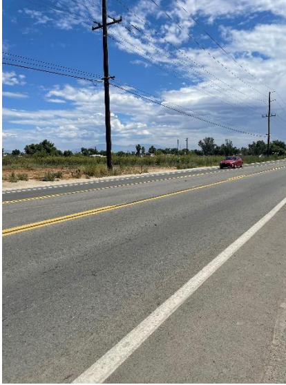
Photo 5: Facing northeast in the BSA.
