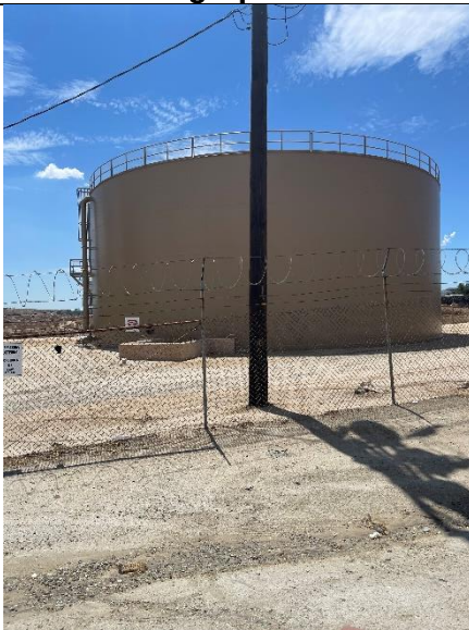
Photo 16: Facing south (staging area)
