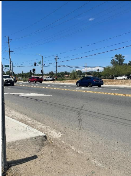
Photo 4: Facing southwest in the BSA.
