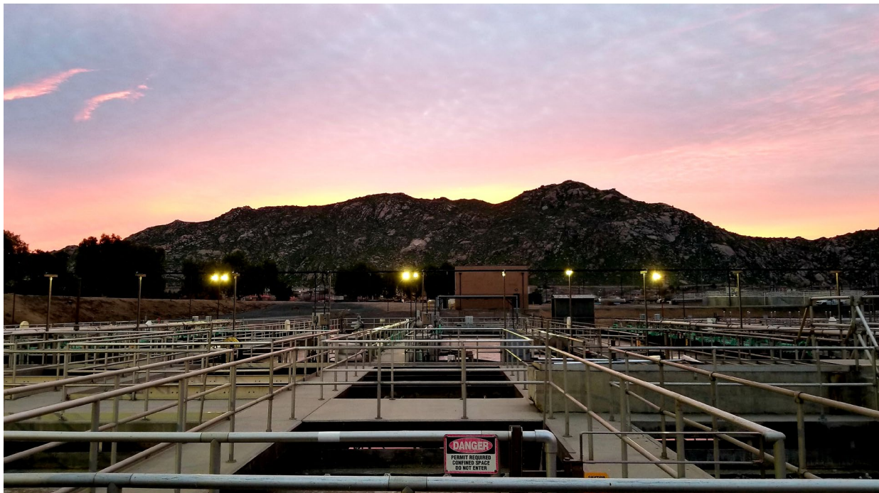
Moreno Valley Regional Water Reclamation Facility
