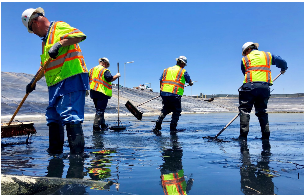
Workers at the Temecula Valley Regional Water Reclamation Facility
