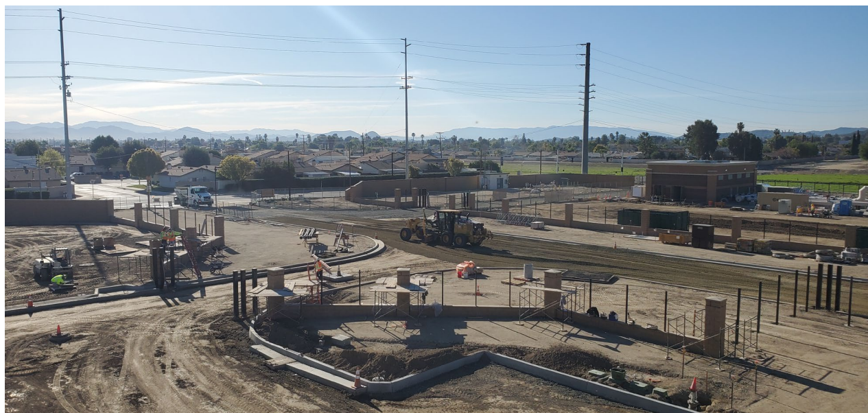
Construction for Desalter Operations
